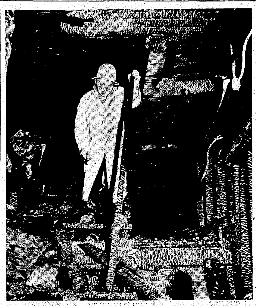
ARSONIST'S WORK: Fire Chief William Fitzgerald examined a back stairway of the Hollywood Hotel, 1607 First Ave., where an arsonist started a fire that took two lives and injured two other persons about 2:08 o'clock this morning. Times staff photos by Larry Dion. (See Page 10 for other photographs.)
